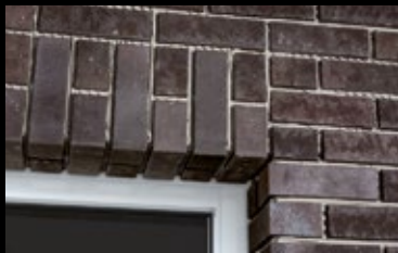
Window lintel perfectly replicated with angles.
