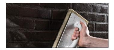
The excess mortar is washed off diagonally with the help of a plaster float with a sponge or foam pad.
