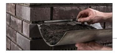
The grouting with a pointing trowel and a metal float in the horizontal direction.
